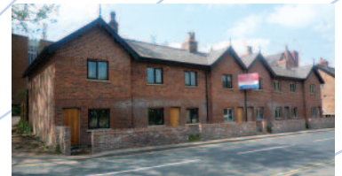
Mill Street, Wilmslow Part refurbishment of 6 houses.
